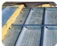
The Roof Hugger retrofit framing system adds a new sloped roof above the existing metal roof. The company produces sub purlins for all existing metal roof profiles that allow re-roofing with your choice of any supplier's new metal panel.
